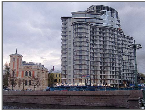
The Monblane luxury apartment building violates existing height restrictions
