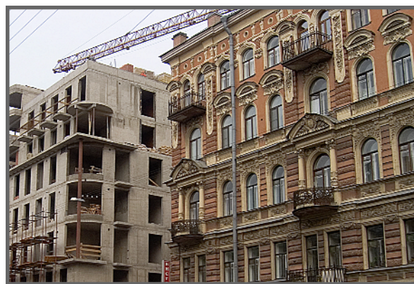
A typical construction scene in the historic center
